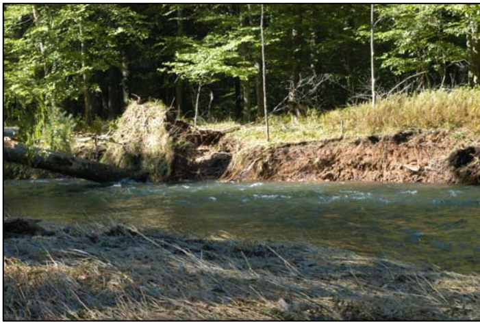
A section of exposed bank to be protected to reduce continuous erosion into the stream. (Courtesy Amidea Daniel, Trout Unlimited)
